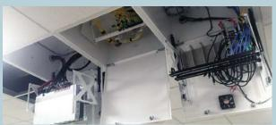
Zone cabling distribution enclosures bring modular flexibility to the point-of-use components specifically designed for space constrained installations in the healthcare environment. These high-density rack-mount enclosures with either adapter panels, ONT's or preterminated cassettes provide for a complete fiber cross connect and patching solution.
